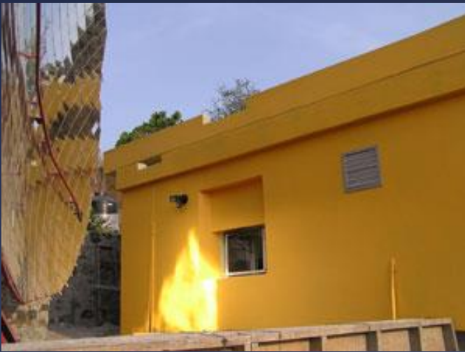
Solar Dish Kitchen – concentrates solar energy to cook food
