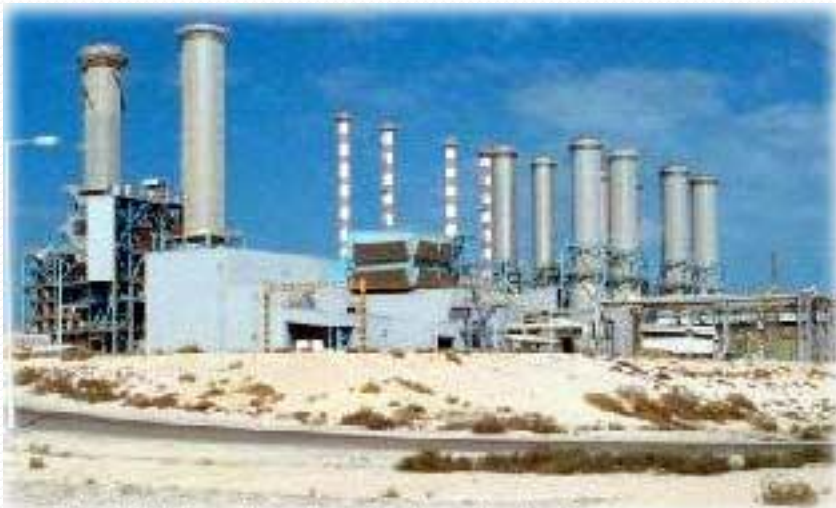
Jebel Ali Desalination Station, Dubai Lahmeyer International
