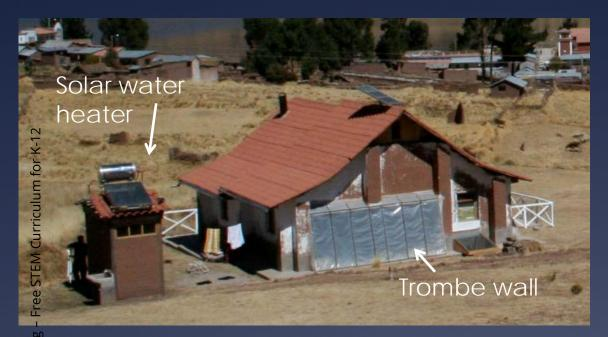
Peruvian home with passive solar heating to beat the home and water , using a Trombe wall and solar water heater
