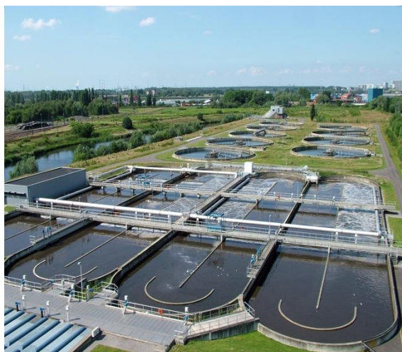
A wastewater treatment facility in The Netherlands.
