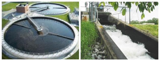
Example secondary clarifier (left), and clean effluent released from a water treatment plan (right).
