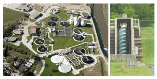
Aerial view of a water treatment plant (left), and example screw pump moving wastewater (right).
