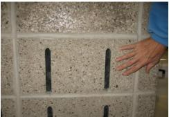
← Lower hallway walls made of concrete masonry units (CMUs) with slots to absorb sound.
