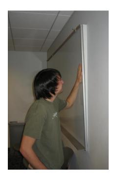
←In a classroom with white boards on all four walls, the boards are tilted at slightly different angles to reduce sound wave reflection within the room.
