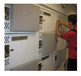
← Fabric and foam locker panels are sound absorbing in a small classroom.
