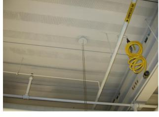
→ Ceiling-floor acoustic decking (metal with many, many tiny holes) placed between the ceilings/floors of the building during original construction minimizes sound reflection in large, open lab spaces.
